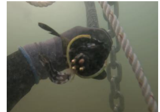
Load cell disconnected underwater
