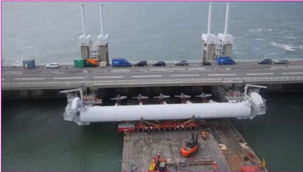
1.25MW dam-integrated array of 5 turbines Eastern Scheldt Storm surge barrier for Tocardo
