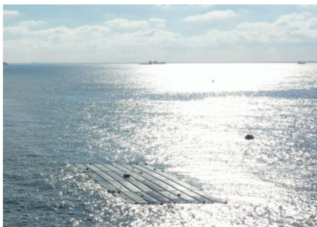
Fig. 3. 200kW offshore floating solar by Oceans of Energy
