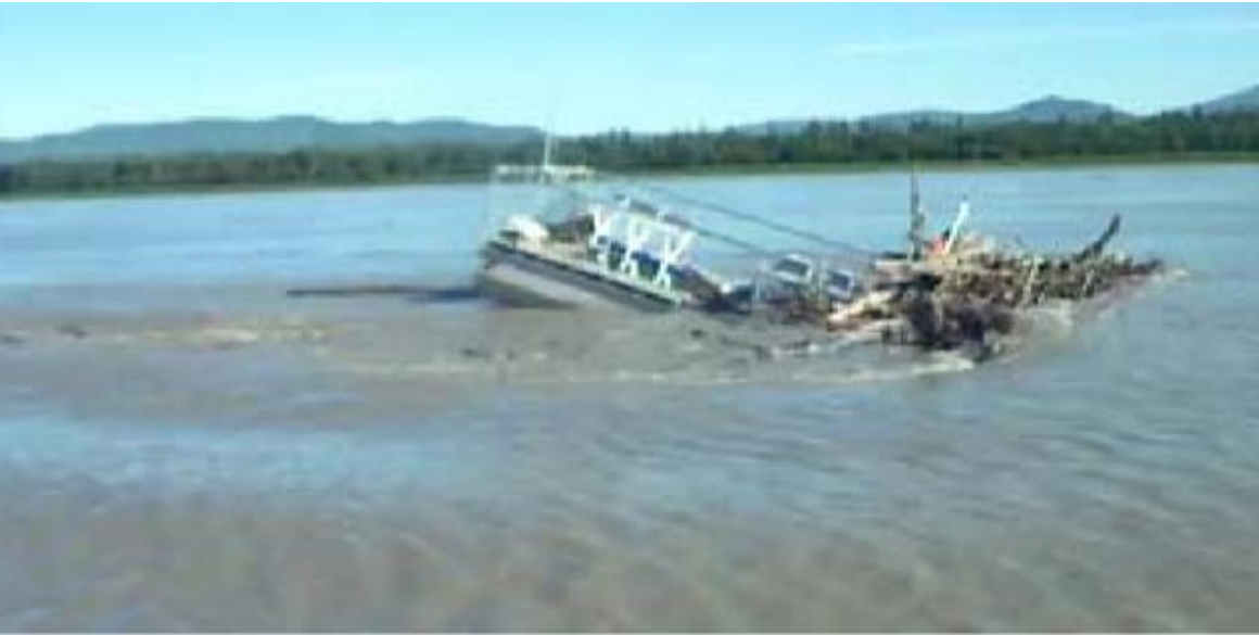
Debris accumulation on surface turbine. Ruby, AK 2013
