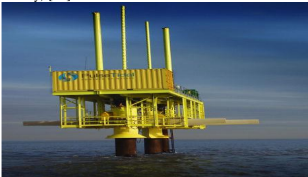
Figure 15a: A complete unit of Pulse Tidal Hydrofoil [42]
