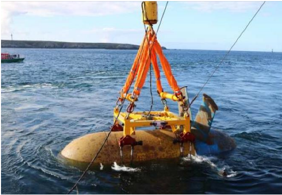
Fig. 12 Launch And Recovery System during turbine's retrieval
