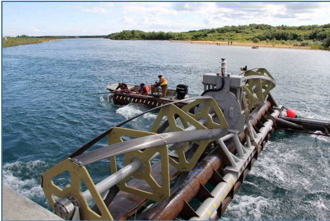
Figure 33: Installing the RivGen® device onto its mooring system, Igiugig, AK, 2015
