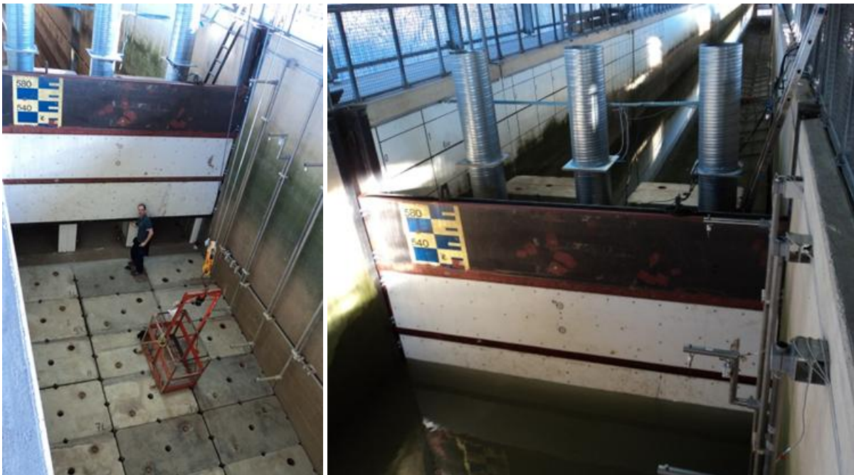
Figure 3: Installation of three OWC caissons in the GWK with 1:6 approach slope, front curtain wall, and three air ducts with orifice plates
