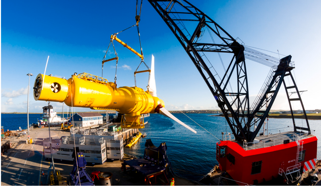
Fig. 5. The DeepGen-IV 1 MW tidal turbine being deployed from Hatson Quay, Kirkwall, Orkney.
