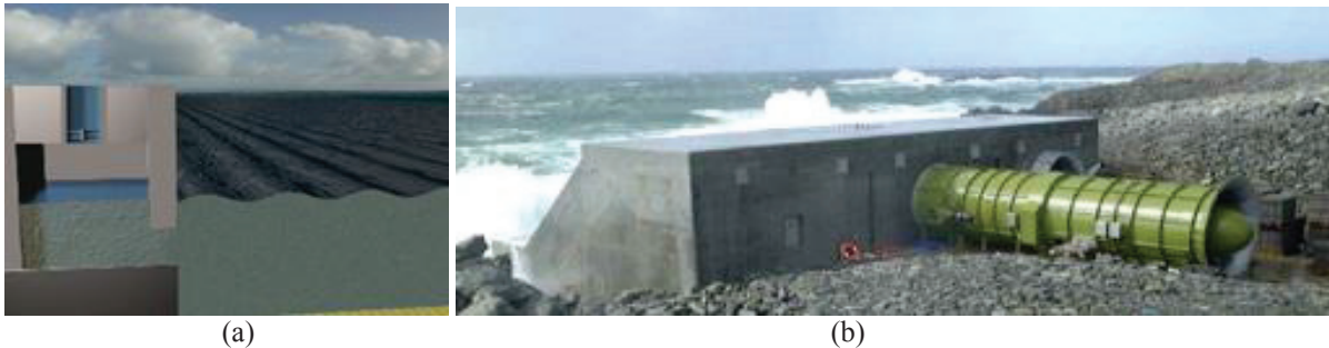
FIGURE 13. (a) Concept of Oscillating Water Column [21] (b) Prototype of LIMPET Constructed In 2000 on the West Coast Of The Scottish Island Of Islay [26]
