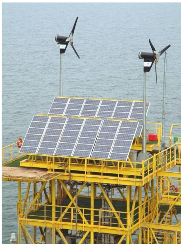
Fig. 1. A prototype of solar and wind energy generator integrated into offshore oil and gas platform (Rosebro, 2006).
