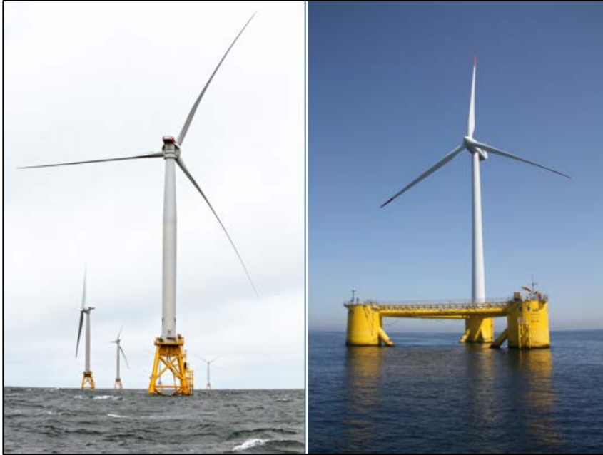
Figure 7. Offshore wind technologies: fixed-bottom foundation (left) and floating foundation (right). Photo Credits: Dennis Schroeder, NREL (left) and Senu Simivas, NREL Image Gallery number 27598 (right).
