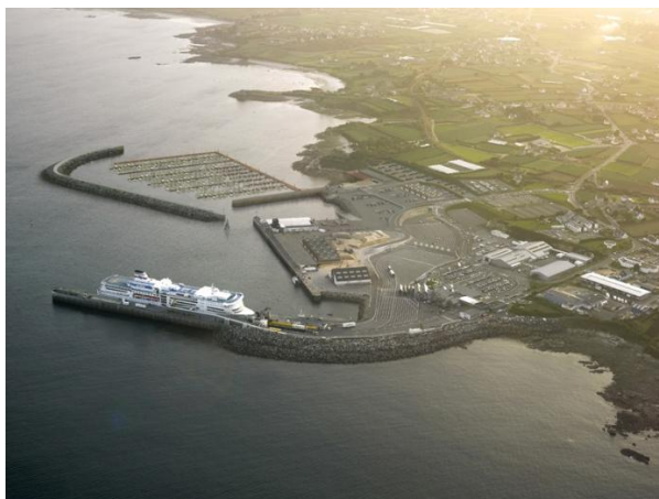
FIGURE 15 : Roscoff port aerial view
