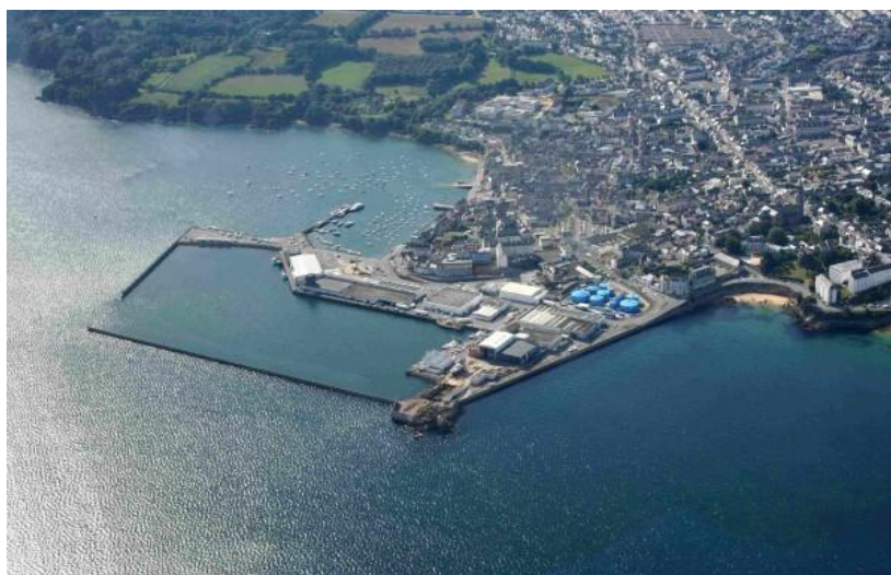
FIGURE 16 : DOUARNENEZ PORT AERIAL VIEW (©GEOMAR)
