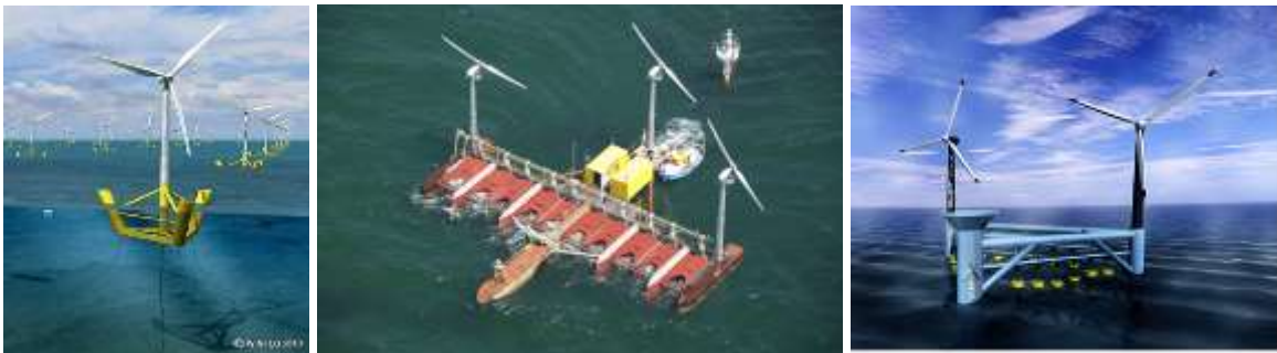
Figure 1: MRE devices with supporting structures ( from left ) artist's impression of WinFlo concept (source: WinFlo), prototype of the Poseidon Floating Power Plant (source: Knud E Hansen A/S) and artist's impression of the W2Power concept (source: Pelagic Power)
