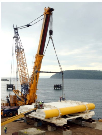
Figure 6: Load-out of Oyster 1 for transport to EMEC
