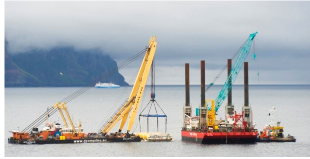
Figure 7: Deployment of the Oyster 1 device at EMEC. Jack-up barge remains after drilling and pile insertion
