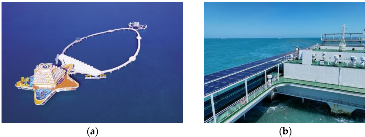
Figure 22. The integration of aquaculture and solar energy: (a) Genghai #1 [142] and (b) Pusheng aquaculture #3 [142].
