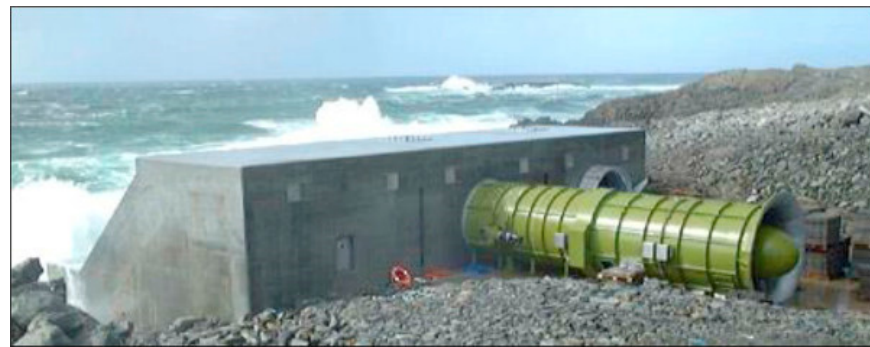
Figure 10. LIMPET OWC plant installed on the island of Islay (Scotland, UK) (Reproduced with permission 5139250512092 from [50], Elsevier, 2016).
