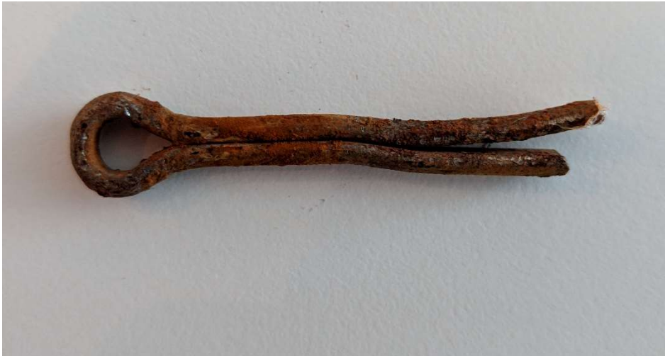
Figure 25 - Cotter pin used in safety shackle. Zinc plating is entirely lost and severe corrosion can be seen.
