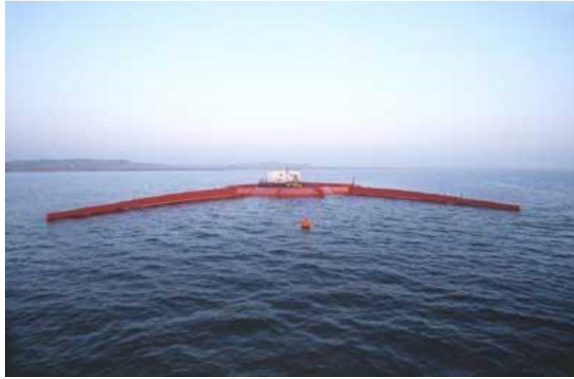
Figure 2: The world's first offshore wave energy converter, the Wave Dragon, is an overtopping device. Waves flow over the top of the device into a reservoir, after which they are funneled through a vertical turbine, creating energy. After the absorption process, the water flows back into the ocean. Image from Wave Dragon.
