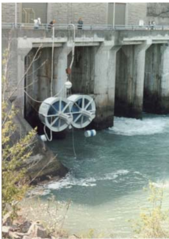
Figure 81 Twin UEK Turbine Installed at Ontario Hydro
