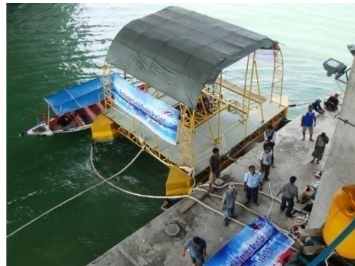
Figure 9. Prototype installed in bridge pillar no. 56
