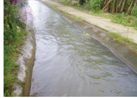
FIGURE 4: Irrigation canal for turbine test.
