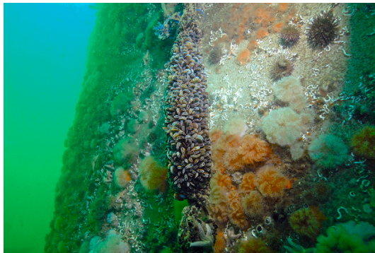
Fig. 2. Biofouling community observed on the foundation of a gravity-based offshore wind turbine in Belgium, including blue mussels, plumose anemones, sea urchins, common starfish, barnacles, and tubeworms [55].
