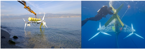
Fig. 5. Deployment and installation of the GEMSTAR prototype at the Renew-MEL laboratory in the Strait of Messina.
