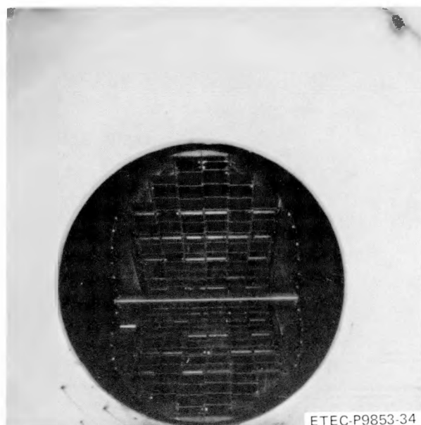
Figure 5-20. Amertap Ball Collection Screen – Catch Mode
