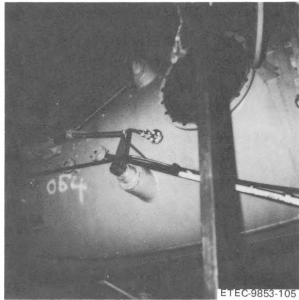
Figure 4-5. Condenser Amertap Unit Showing Pressure Taps
