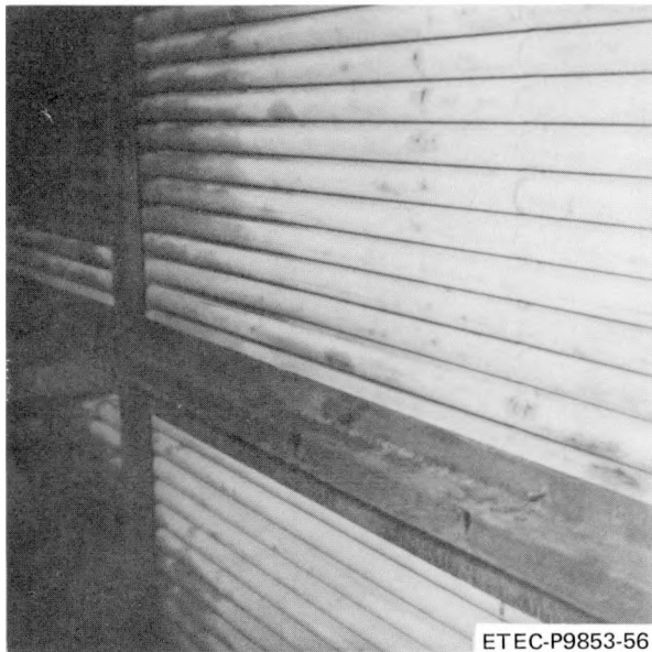
Figure 5-40. Evaporator Enhanced Tubes Looking Aft, Starboard Side
