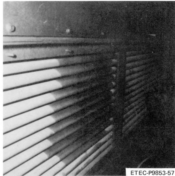
Figure 5-41. Evaporator Enhanced Tubes Looking Forward, Starboard Side
