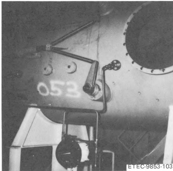
Figure 4-4. Evaporator Amertap Unit Showing Pressure Taps
