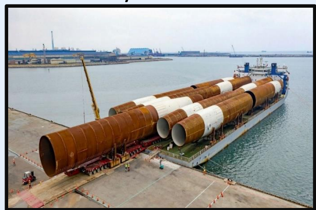
Fig. 2. Monopiles for Taiwan's Formosa 1 offshore wind farm.
