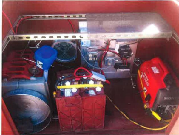
Figure 2: Box setup: Fuel supply to the left, Fan in the back left, Batteries in the front, Power electronics on the back panel, Generator on the far right.
