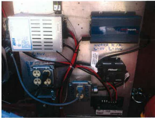
Figure 3: Power panel setup: Top left: Battery charger and controller (small black box on top); Top right: DC-AC inverter; To the left: 13 A 115 V outlets and AC power on/off switch; Right: 150 W 115 V AC outlets; Bottom Right: SunSaver Solar Charge Controller.
