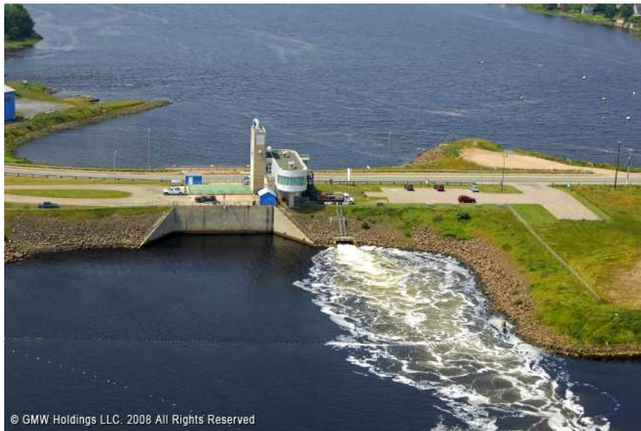
Figure 16 Annapolis tidal power plant [26].
