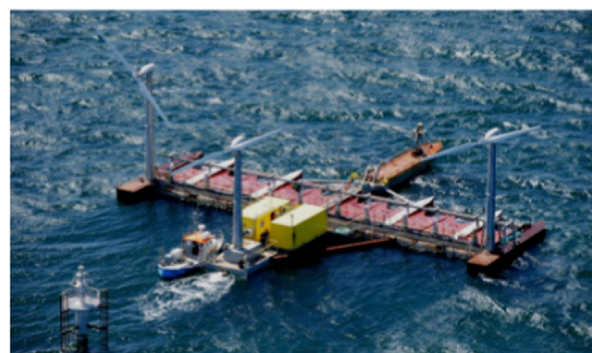
FIGURE 7 Poseidon floating power system integration of wind and wave energy (TETHYS, 2014)
