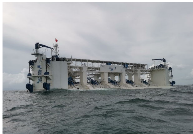
Figure 2. The megawatt-scale floating WEC, Nankun.
