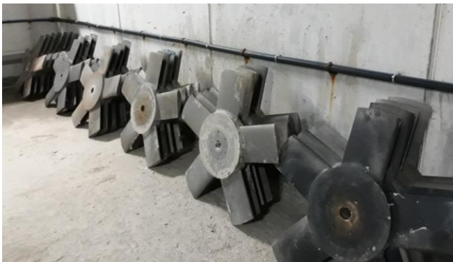
Figure 11: Replaced Wells turbines in Mutriku Wave Power Plant.
