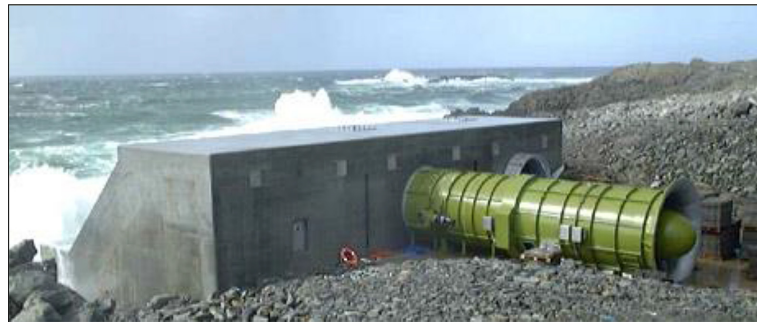
(a) The Limpet WEC device (Heath et al., 2001).
