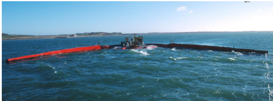
Figure 2.6: The terminator type Wave Dragon WEC (Kofoed et al., 2006).
