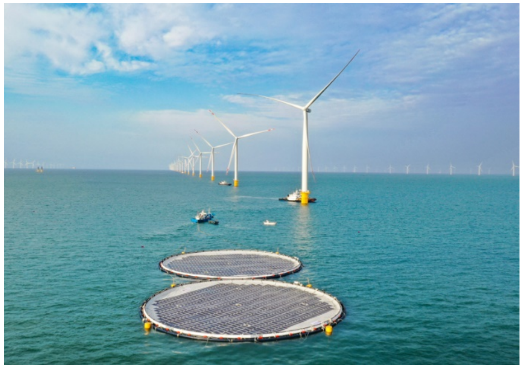
Figure 1. China's first offshore floating PV station using ocean sun floats (water depth: 20–30 m).
