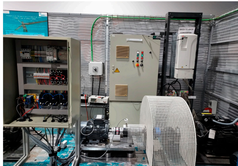
Figure 8. General view of the test bench.
