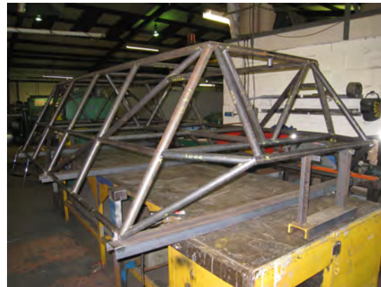
(b) Top Frame fabrication
