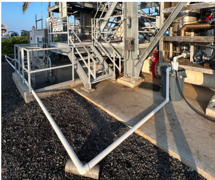
Figure 10. Flushing the ammonia line between the feed pump outlet and recirc pump inlet did not remove significant amounts of shavings/debris.
