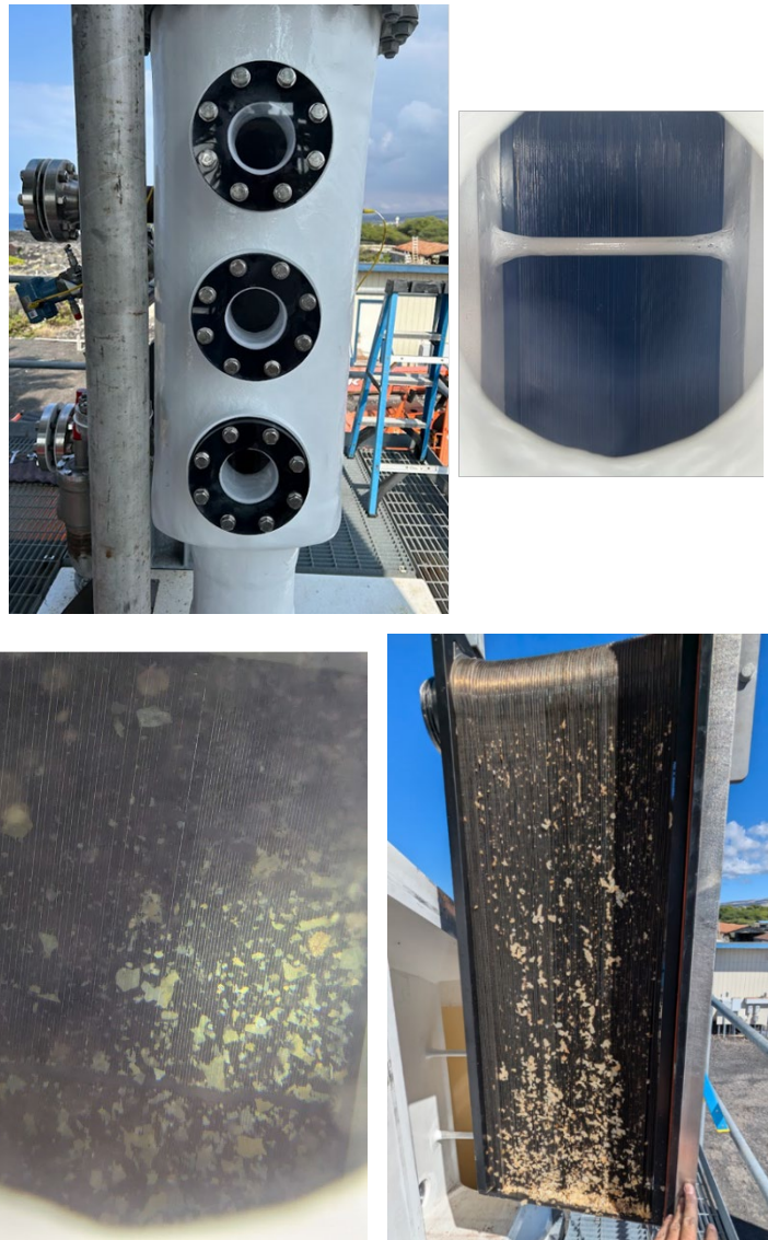
Figure 12. (top) View ports installed to monitor evaporator leading edge. (bottom) Debris from seawater piping system collected at the evaporator leading edge as seen through the viewport and when evaporator was removed for cleaning.
