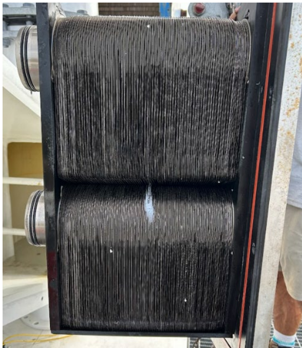
Figure 13. White residue at the center of the stack is indicative of an ammonia leak.
