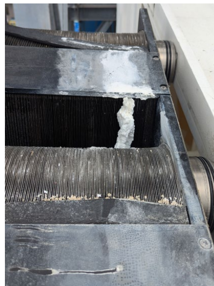
Figure 15. TFHX evaporator showing residue from ammonia leak and debris around the manifolds.
