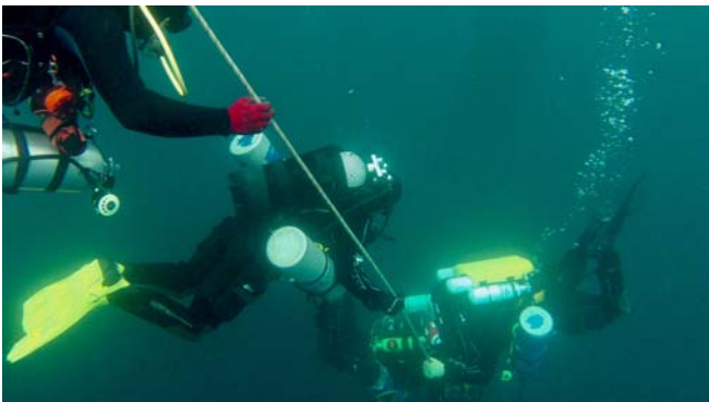
Fig. 7 Ground wire rope replacement operation
