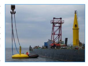
patented three phase, permanent NdFeB magnet, linear generator uniquely developed to be utilised in ocean bed arrays and directly driven by point absorbers on the ocean surface. The WECs form part of an integrated wave energy power generation system capable of delivering Grid Code compliant power to the on-shore grid.
