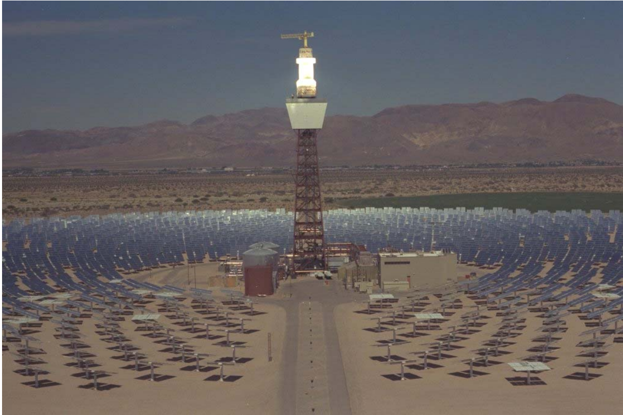
Figure 7-3 Solar Two Central Receiver in Operation. The two tanks to the left of the tower base are the storage tanks for the hot and cold molten salt solutions.
