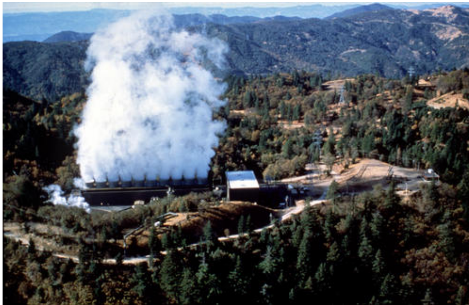
Figure 6-3 Hydrothermal Power Plant at The Geysers, California
