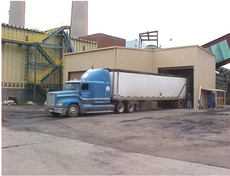
Figure 4-23 Receiving Sawdust at the Willow Island Generating Station
