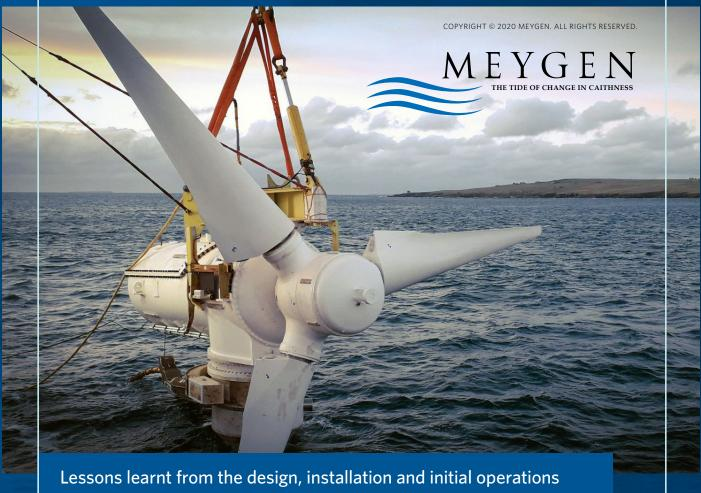
phases of the 6MW 4-turbine tidal array in Scotland's Pentland Firth
