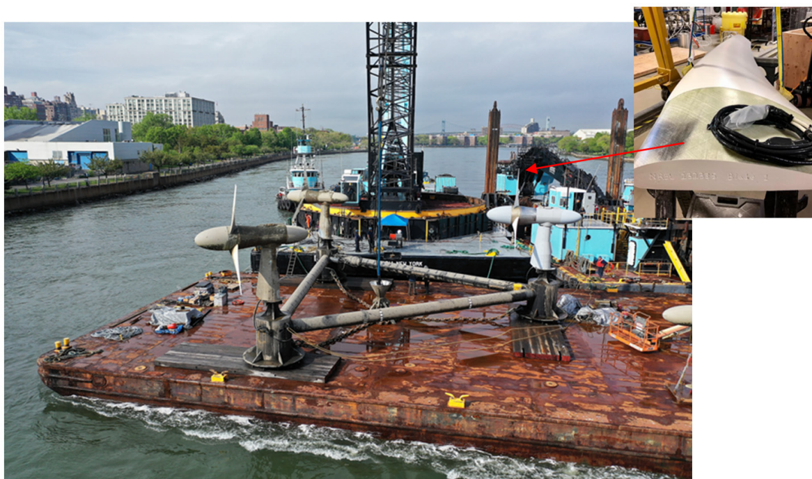
Figure 1. Verdant Power's TriFrame being deployed in the East River in New York, with the National Renewable Energy Laboratory's (NREL's) thermoplastic blades on the turbine in the right side of the photograph. A close-up photograph of one thermoplastic blade is shown, indicated by the arrow.
