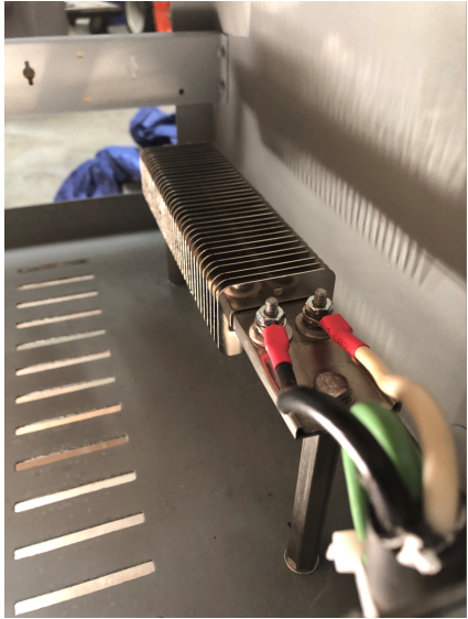
Figure 3.9: [Left] Strip heater installed in resistor bank enclosure. [Right] Dump load resistor bank installed on platform.
