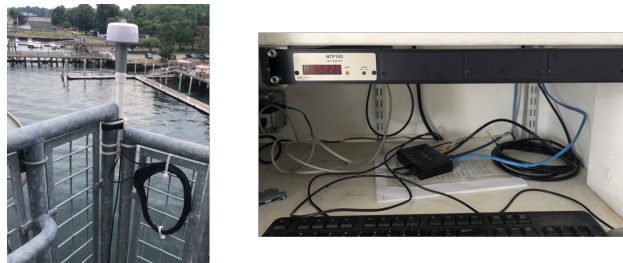
Figure 3.1: [Left] NTP GPS receiver installed on stairwell leading up to Memorial Bridge Control Room [Right] NTP Server installed in the server room located on the Memorial Bridge deck level
