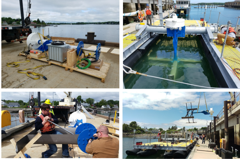
Figure 2.3: Initial turbine assembly and installation (Gagnon 2018, Figure 7.9 [6])
