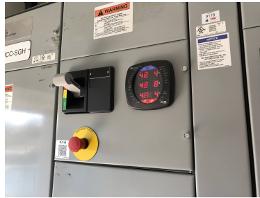
Figure 4.15: The Shark meter installed in the Memorial Bridge Motor Control Center (MCC) 480VAC breaker panel that feeds the TDP
