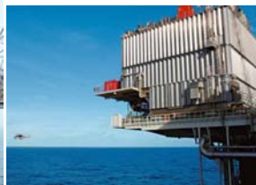
HVDC Light Module on Troll-A platform (ABB)
