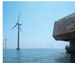
Transformer unit (33 kV/132 kV) for the aggregation of the 72 wind turbines of the park, 165 MW
