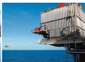
HVDC Light Module on Troll-A platform (ABB)
