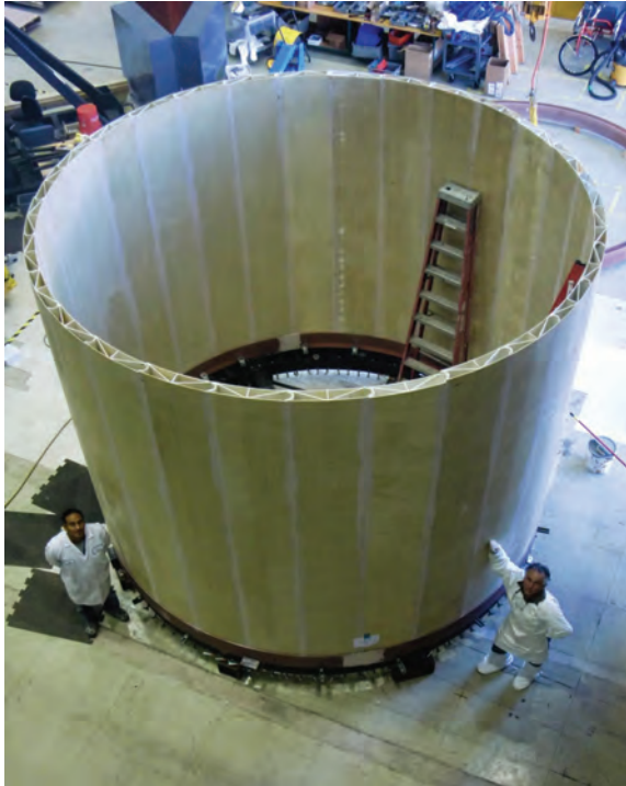
Figure 1. The first assembled core ring for 4 m diameter CWP. Note the size of the core ring compared to the two persons in the photo. Photo taken by the author.
