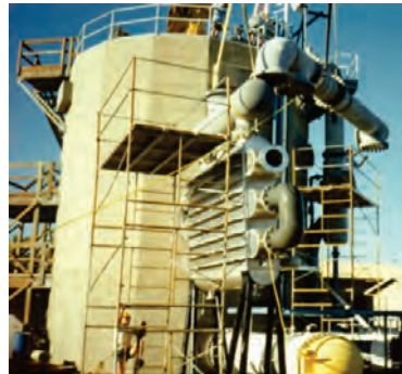
Figure 2. 210 kW Open-Cycle Pilot Plant with Surface Condenser for Water Production. Photo by the author.
