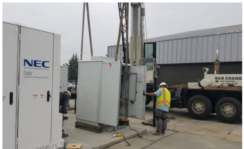
EWEB contractor installs back-up battery power system.
