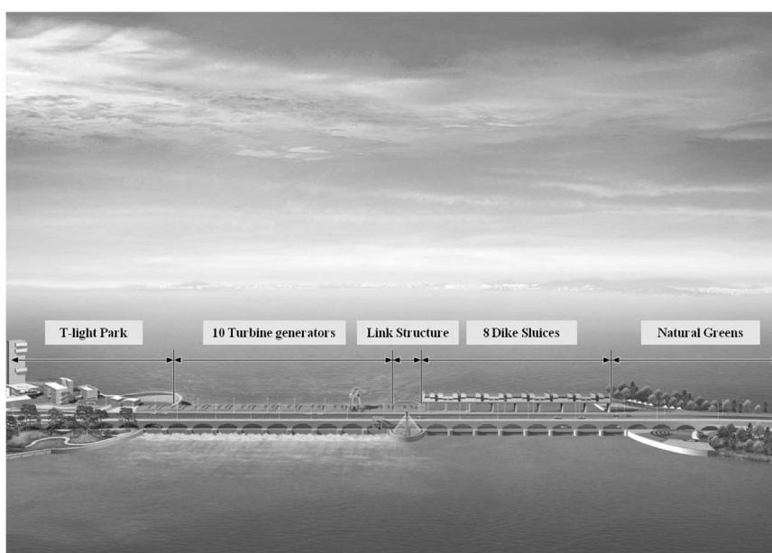
Fig. 6. Overview of the Shihwa tidal power plant.
