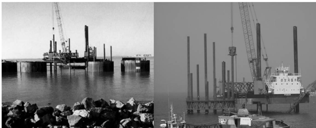
Fig. 15. Circular cell temporary cofferdam construction by SEP barge.
