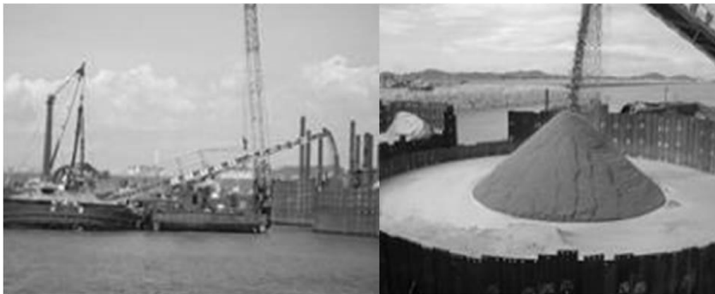
Fig. 13. Circular cell sand filling.
