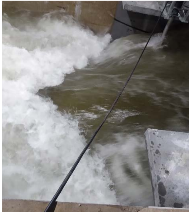
Figure 17. Turbine on the edge of under-submergence
