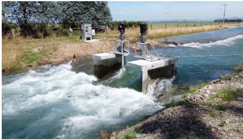
Figure 3. Emrgy Turbine Installed in Canal
