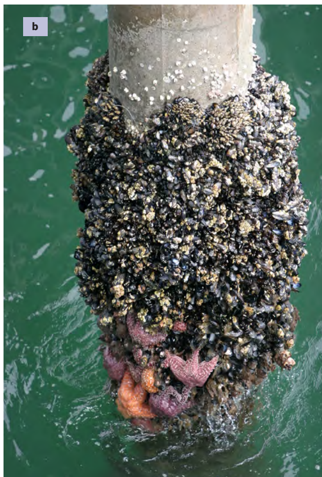
Figure 2.4 a) A concrete marine structure with severe biofouling. Source: Vorathep Muthuwan /Shutterstock.com; b) Mussels on a pier pillar. Source: Mikeledray/Shutterstock.com
