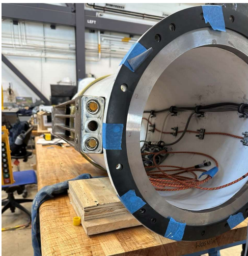
Fig. 9. Cooling radiator installed on the generator housing at turbine back nacelle section.
