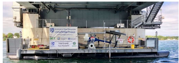
Fig. 12. AMEC-UNH Tidal Energy Test Site at Memorial Bridge, Portsmouth, NH, USA [18]
