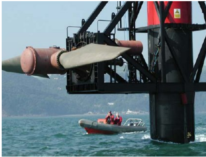
Figure 5-4: The SeaFlow demonstration plant near Devon, UK [53]
