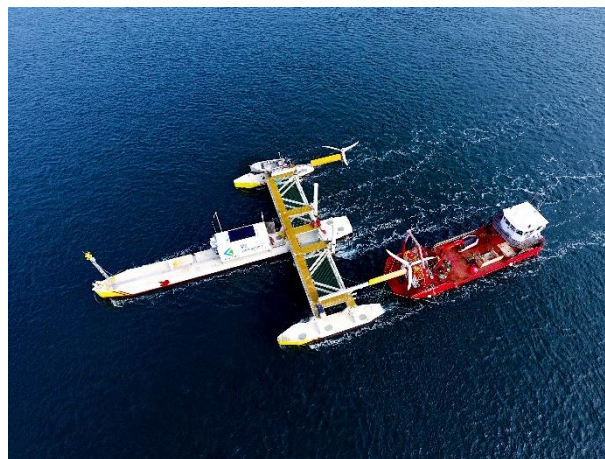
Fig. 2 Blade installation (6.3m rotors) in Grand Passage
